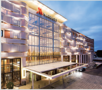
Marriott Auditorium Hotel, Madrid, Spain
