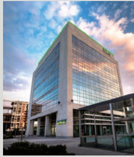
HQ Mansion of DKV, Spain
